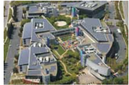
Decentralized solar power plant on the rooftop in California
