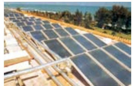
Figure 4 Solar water heating for hotel industry Installed at Hotel Fisherman's Cove (Taj Group), Chennai
