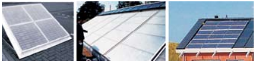
Practical examples of PVT devices: glazed PVT liquid module, glazed PVT liquid system RES ( www.beaufortcourt.com ), unglazed PVT air roof
