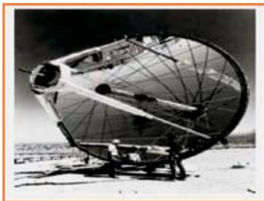
Figure 6 300-kilowatt linear concentrators. (Tom Lances - Austin American Statesman/PIX00014)
