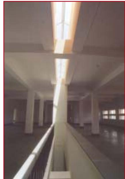
▲ The skylight on the roof of West Bengal Renewable Energy Development Agency office building provides natural light for inner office spaces and is connected to the office spaces for inducing ventilation by stack effect
