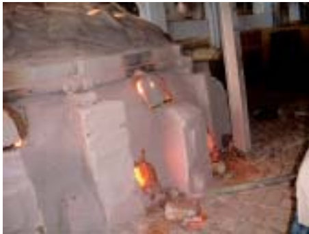
(i) Dismantling of pot furnace wall begins
