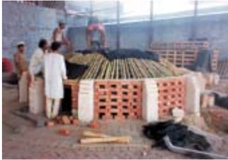
(iii) Filling the structure with mud
