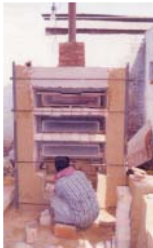
(iii) 3-tier version under construction
