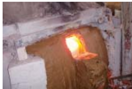
(xii) Completed wall
