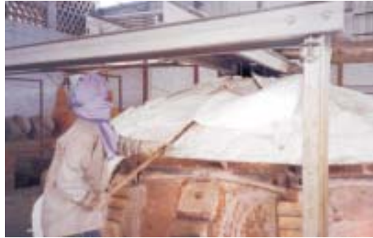
Figure 33 Ceramic fibre being laid on the crown
