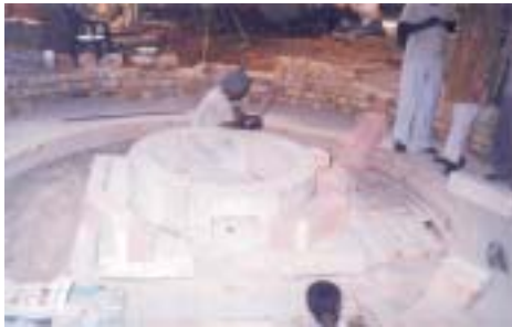
(i) Circular Zirmul block being laid for central well
