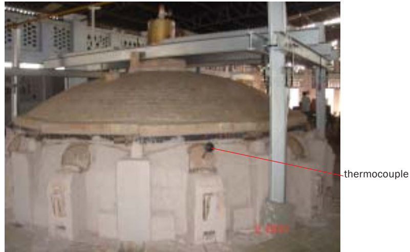
Figure A2-1 Measuring furnace temperature
