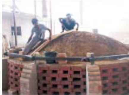
(iv) Using a wooden leveller to give a uniform curvature
