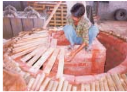
(ii) Using bamboo and planks as support
