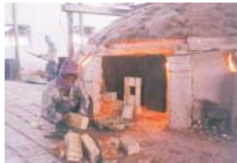
(x) Rebuilding of wall begins with placing of the centre piece
