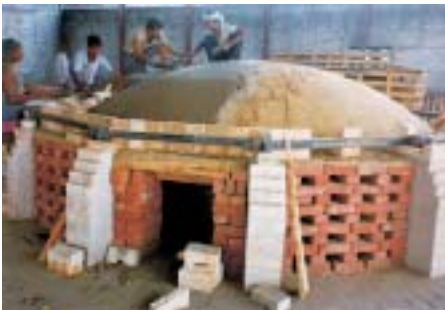
(v) Plastering the crown with mud
