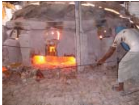
(ii) Dismantling of wall progresses
