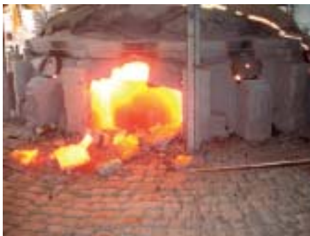
(iii) Wall dismantled, showing failed pot inside furnace
