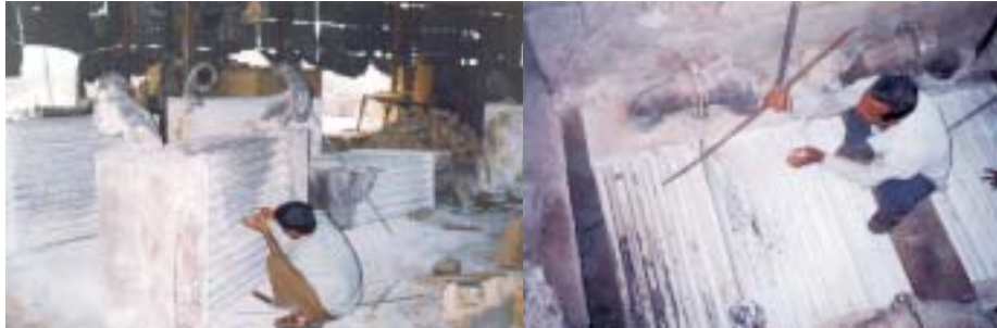
Figure 34 Cleaning the recuperator modules
