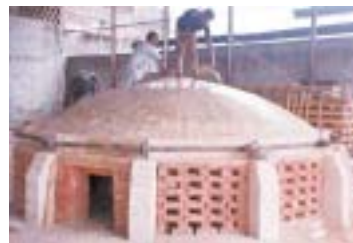
(viii) Washing the crown with silica mortar
