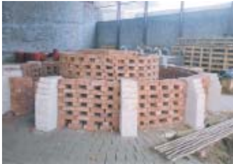
(i) Making a concentric red brick structure
