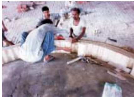
(vi) Fixing silica bricks
