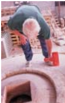
(vii) Lee tests the key brick
