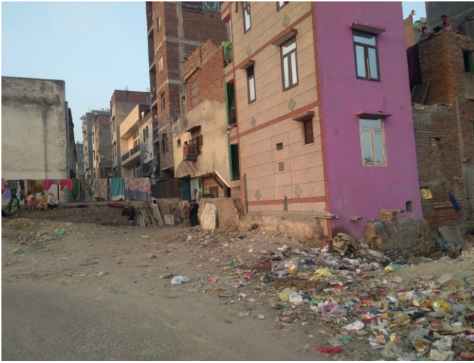
Figure 6 Section of an unplanned (informal) residential colony (Haji Colony) near the Okhla waste-to-energy plant
