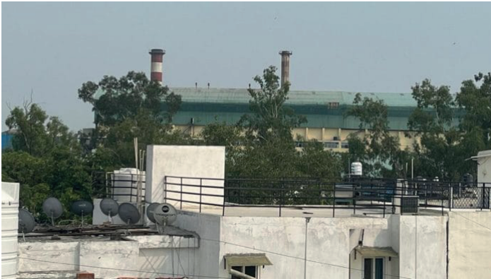
Figure 7 Okhla waste-to-energy plant as seen from the roof of a house in Sukhdev Vihar
