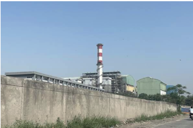
Figure 5 Waste-to-energy plant in Okhla, New Delhi
